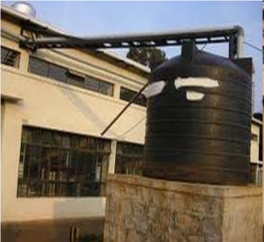
Alternative source (Rainwater Harvesting)
